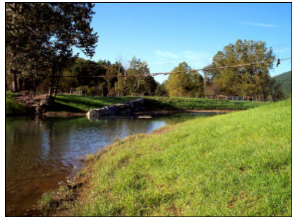
Photo 5, Post-construction: View looking downstream at the same channel as in Photo 4. Note the restored streambank with vegetation and rock vane to protect the bank from future erosion. A new meander was created just beyond the rock vane where the channel had previously been straightened.
