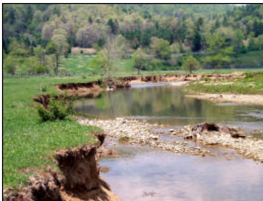
Photo 1, Pre-construction: View is looking upstream at the starting point for Site 24. Note the eroding banks, excessively wide and shallow channel, and deposition of mid-channel bars.
