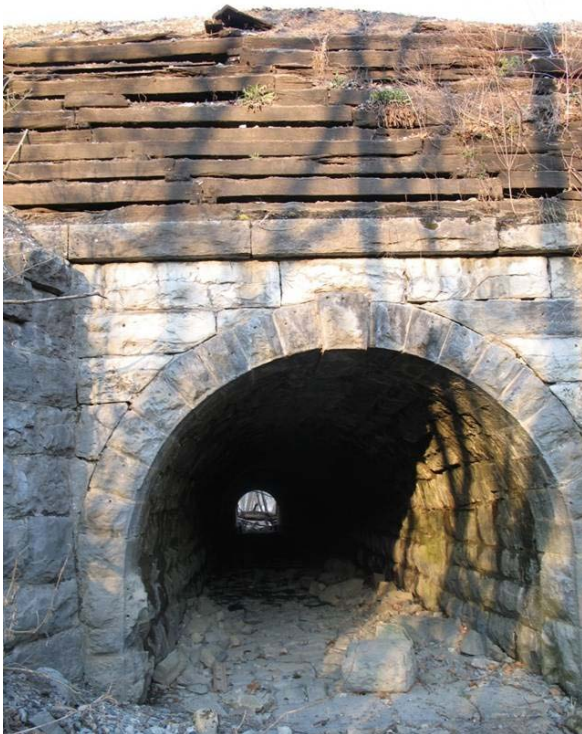
Figure 3: Storm water tunnel
